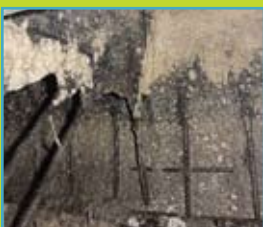
Exposed re-bar (left and middle) on a 5-year-old concrete interceptor and interior collapse (right) in a 6-year old concrete interceptor.
