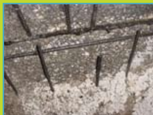
Exposed re-bar (left and middle) on a 5-year-old concrete interceptor and interior collapse (right) in a 6-year old concrete interceptor.
